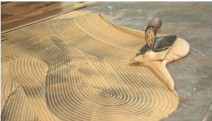
Silane-terminated polyurethanes (STP / **Desmoseal® S**) combine the advantages of a polyurethane backbone and a silane-based curing mechanism. Therefore STPs provide a unique combination of excellent cohesive strength and good adhesive properties.
